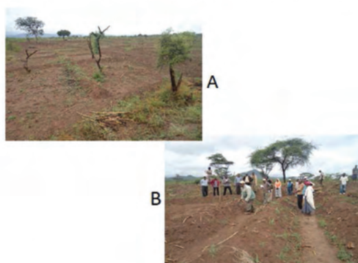
Figure 55: Water harvesting structures within plots at the Segen Irrigation project (A) and Arba Minch Diocese EECMY-DASCC irrigation project head Mr Galunde showing the diversion (B)
